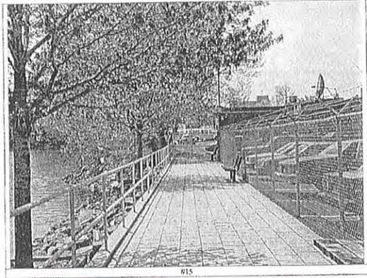
Isolated Section of Existing Walkway
