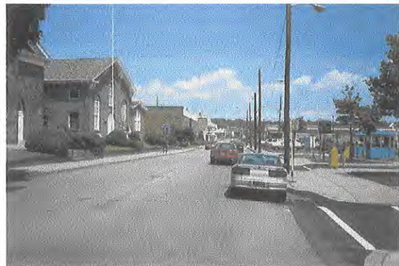
Court Street Looking East. Notice Curb Cuts and Parking on Right
