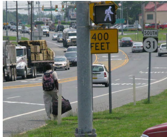
Lack of a sidewalk network, particularly along busy roadways, creates difficult and unfriendly conditions for pedestrians.
