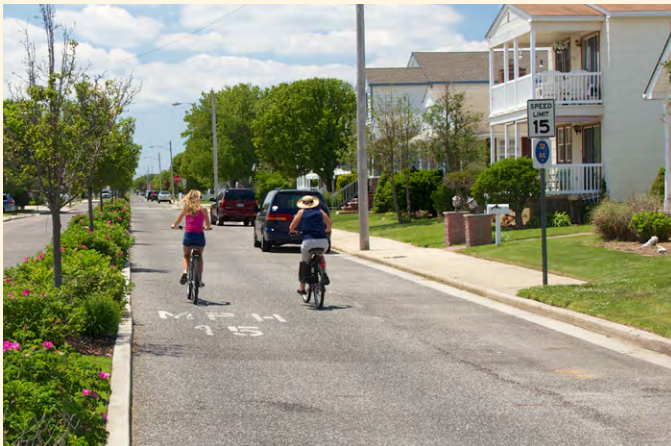
Bicycle boulevard on Haven Avenue in Ocean City, NJ, has a 15 mph speed limit and uses curb extensions and a raised median to slow traffic and reduce cut-through traffic.
