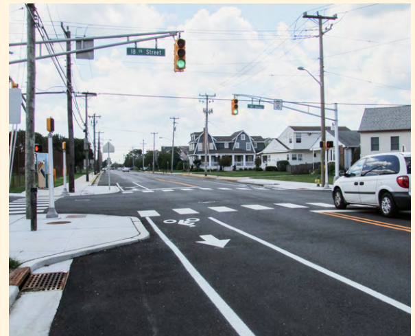
Road diet implemented on CR 656 in Ocean City integrates bicycle lanes and curb extensions.
