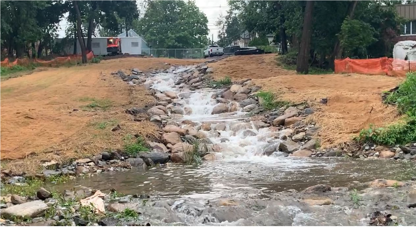
Stormwater Canyon After
