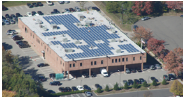
Figure 1. Solar panels on Bergen County facility (Courtesy of Solar Energy Directory).
