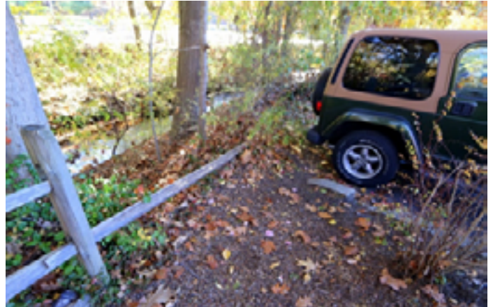
Figure 7. Without interventions to capture runoff, impervious surfaces can drain directly into adjacent water bodies.
