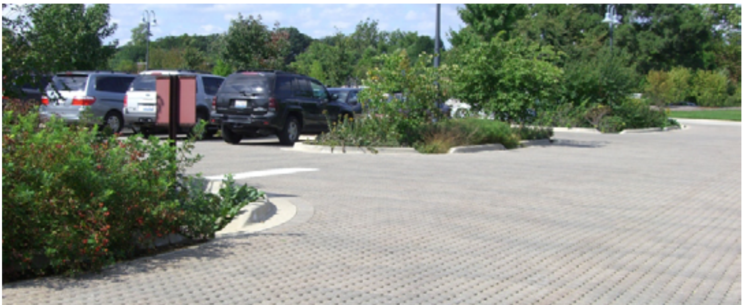
Figure 22. Implementing stormwater best management practices, like the parking lot rain gardens above, can protect and enhance the ecological health of natural resources in the parks, as well as improve user experience (Courtesy of Biohabitats).
