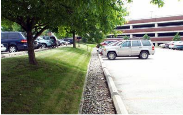
Infiltration beds in a parking lot
