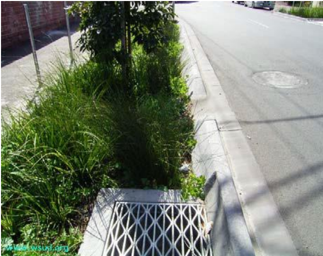
Bioretention swale retro-fit to roadway
