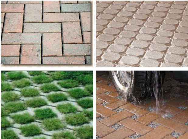
Permeable paving options
