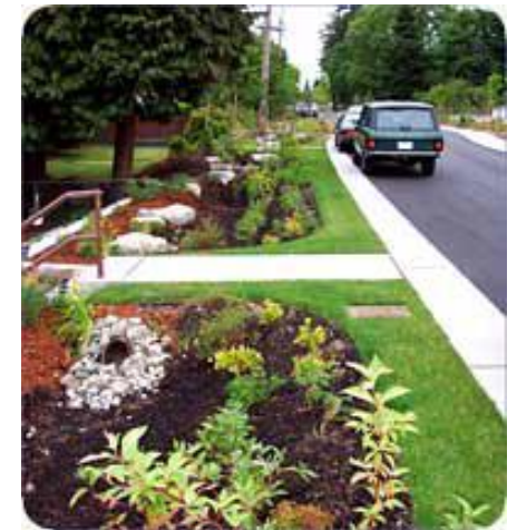
Bioswale along a Residential Street
