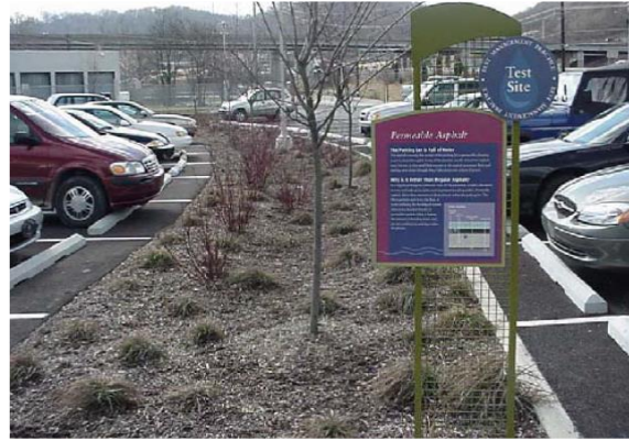
Bioretention swale in a parking area
