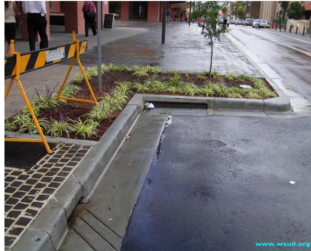
Street tree stormwater treatment retro-fit
