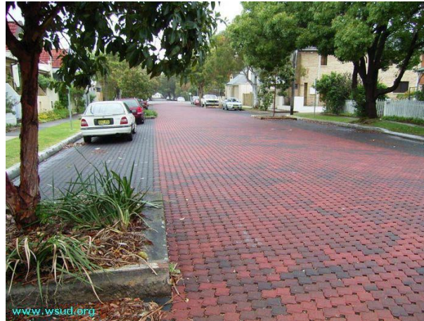
Permeable paver retro-fit for a residential street
