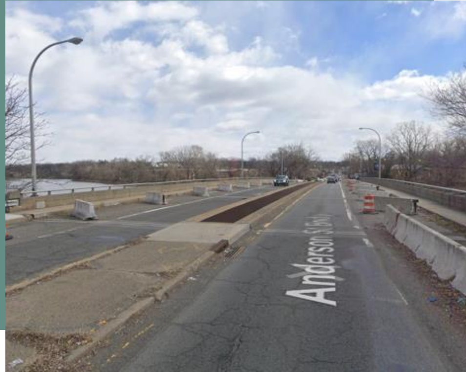
Anderson Street Bridge
