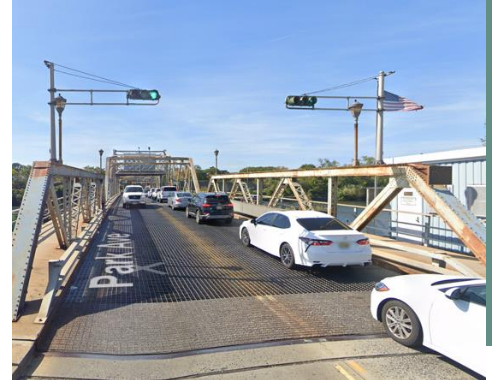
Kingsland Avenue Bridge
