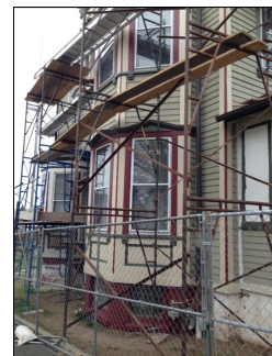
Bianchi House during restoration.
