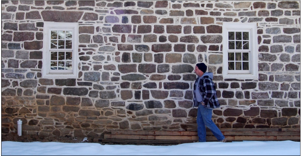
Tim Adriance on the job at the Terhune- Demarest Dwelling House, Ho-Ho-Kus.
