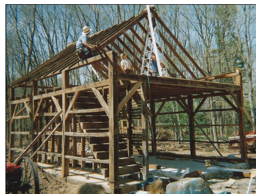
Below: Reconstructing "new barn" on old original foundations
