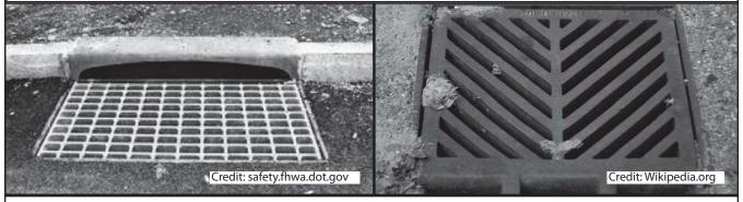
Bicycle-safe drainage grates typically cost \$450 each for a 2'x3' unit.
