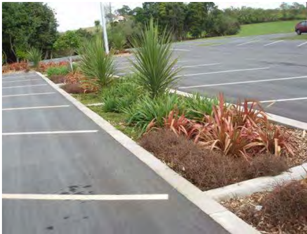
Rain Garden in Parking Lot
