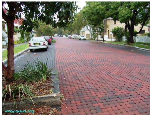
Permeable paver retro-fit for a residential street
