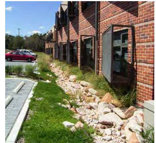
Permeable parking lot and bioretention system for commercial buildings
