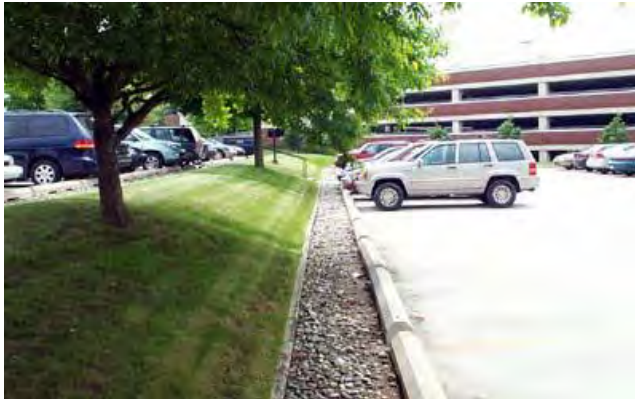
Infiltration beds in a parking lot
