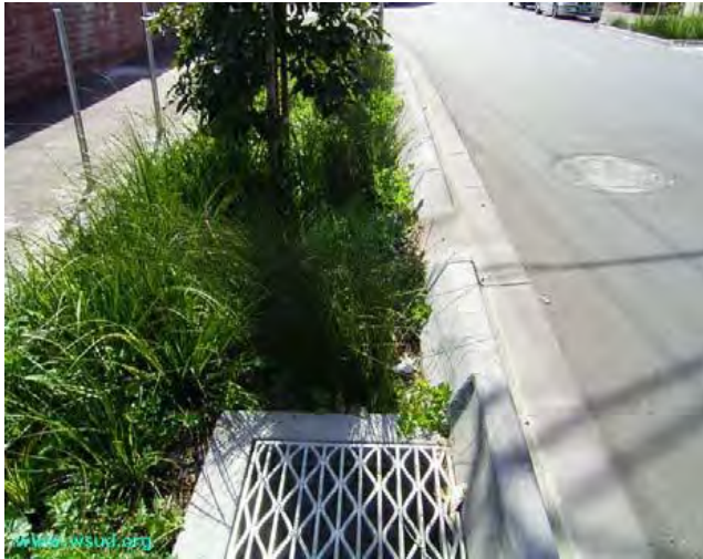
Bioretention swale retro-fit to roadway
