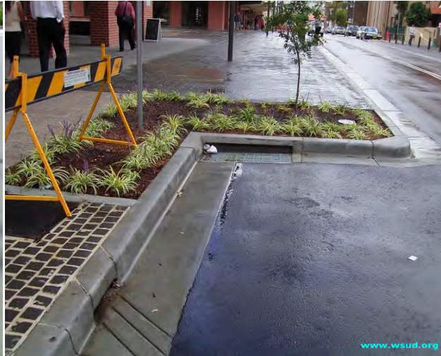
Street tree stormwater treatment retro-fit
