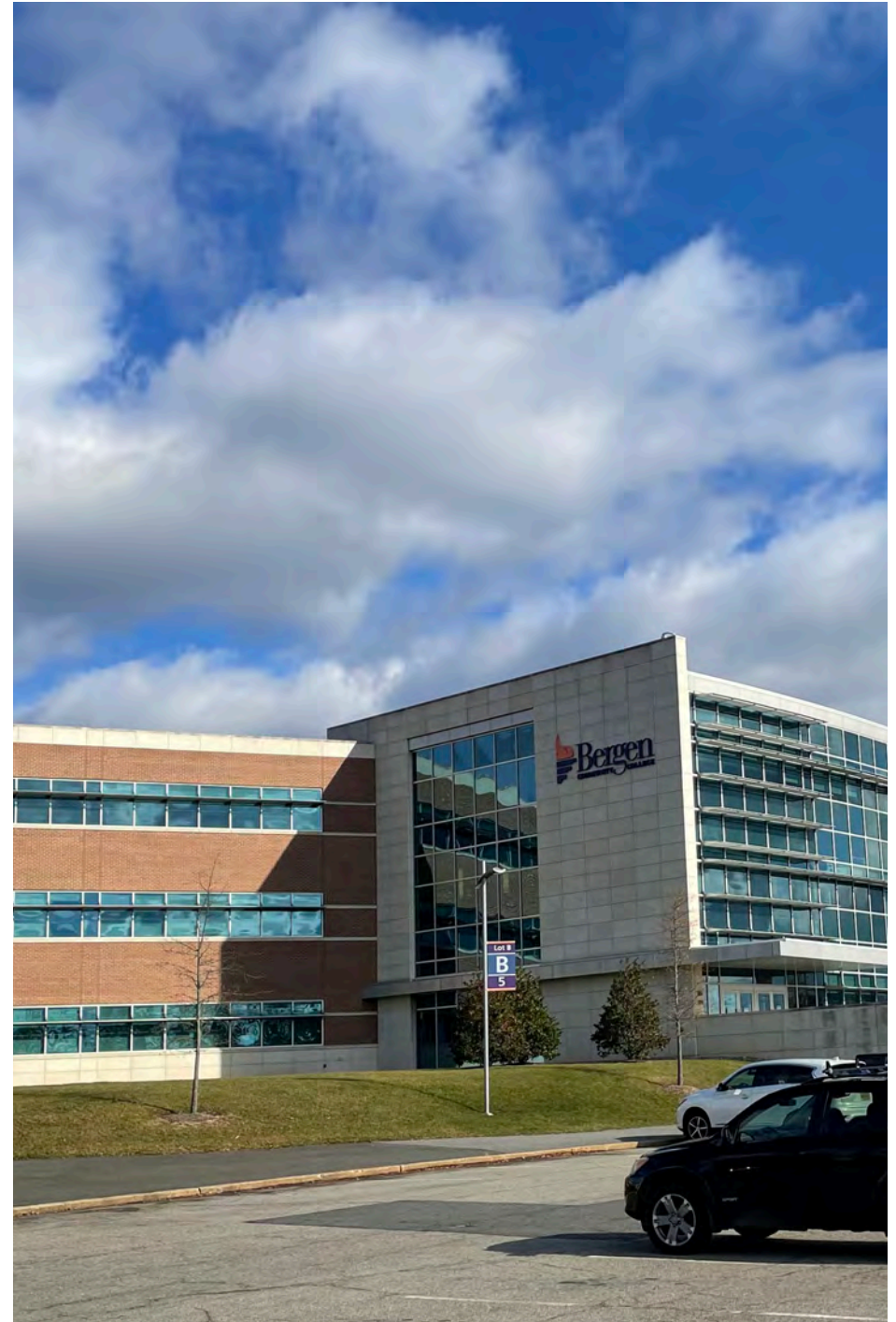
Bergen Community College. Source: Colliers Engineering & Design
